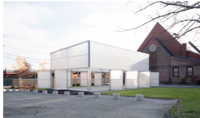
Southside Cultural Center of Rhode Island Photo by Naho Kubota, photo courtesy of Ultramoderne
