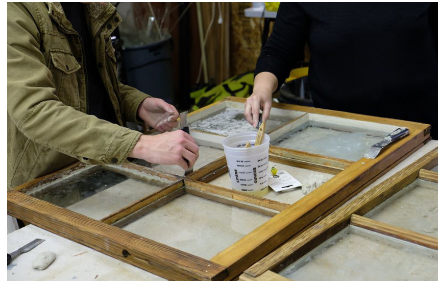
Students participate in a window repair workshop as part of their curriculum; photo courtesy of Clatsop Community College Historic Preservation and Restoration Program
