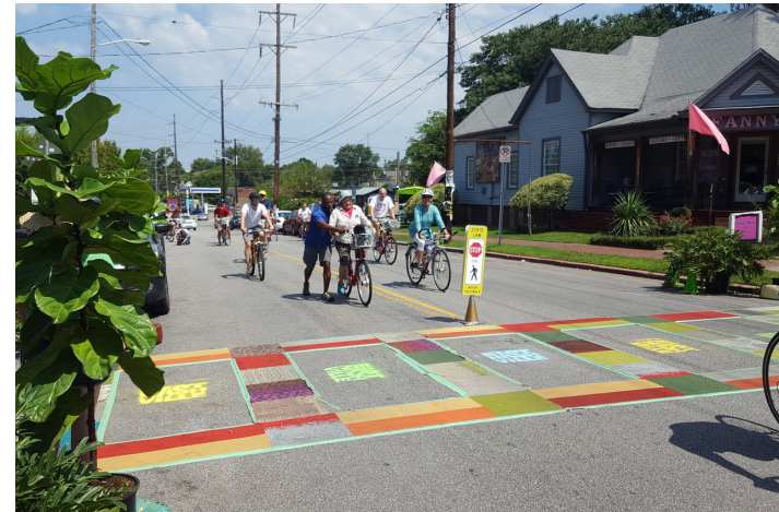
Tactical urbanism in Nashville, installing a temporary crosswalk at a busy intersection; photo courtesy of Nashville Civic Design Center
